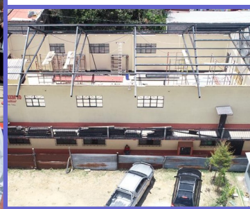
New roof for Sumpango church
